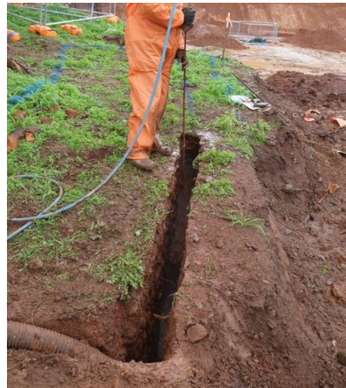
Less damage is done to tree roots if utilities are tunneled under a tree (left, top and bottom) rather than across the roots (right, top and bottom).
