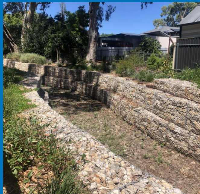
Rock filled gabions
