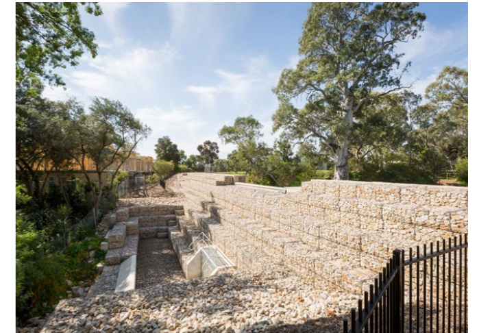
Flood Control Dam
