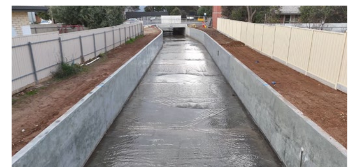
Channel construction through to completion
