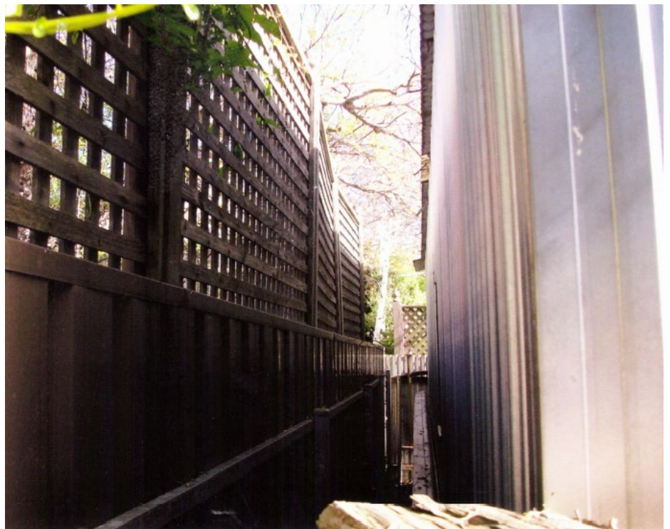
Space between existing outbuilding and subject boundary fence at 61 Dover Street.
