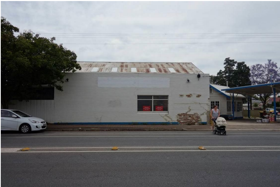
Side wall of the former workshop building viewed from Duthy Street
