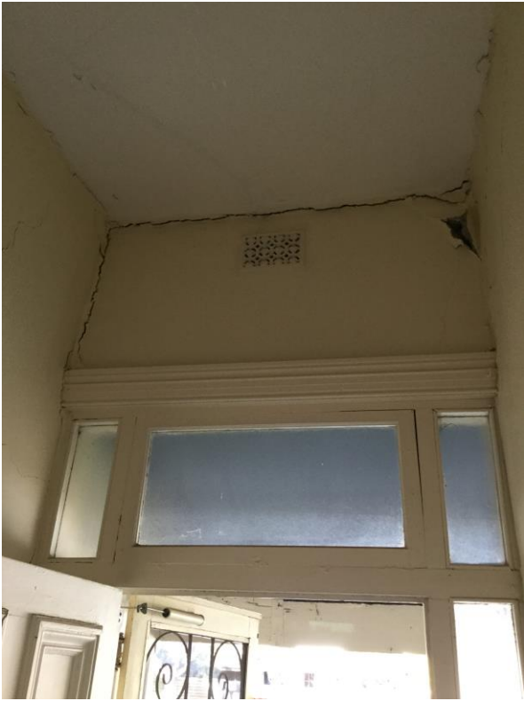
*Inside, above front entry doorway
