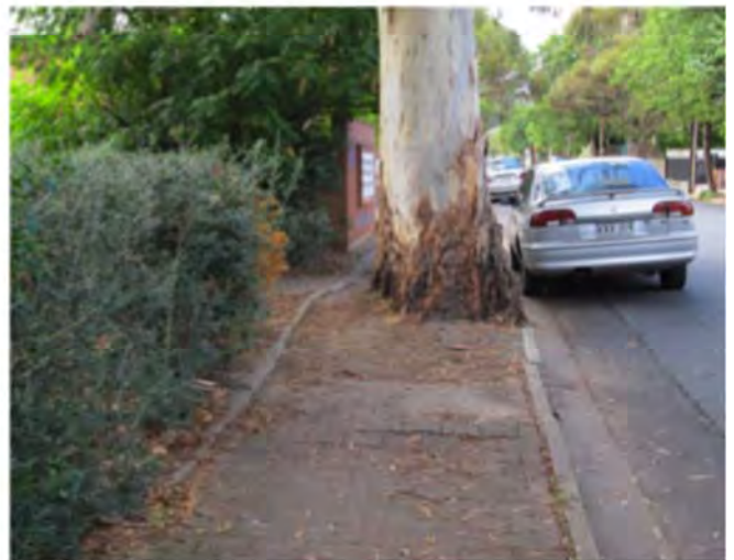
Example in Mary Street, Unley where footpath width narrows due to tree trunk. The challenge is to decide if the tree remains or the need for a legislative age friendly footpath takes priority.
