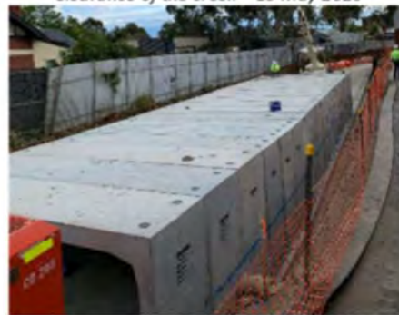
Culvert installation – 20 May 2020
