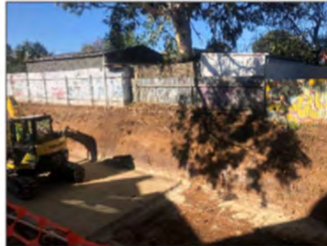
Clearance of the creek – 15 May 2020
