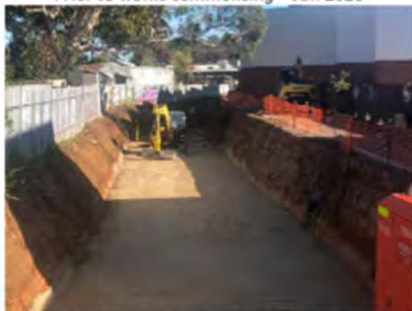
Clearance of creek – 15 May 2020
