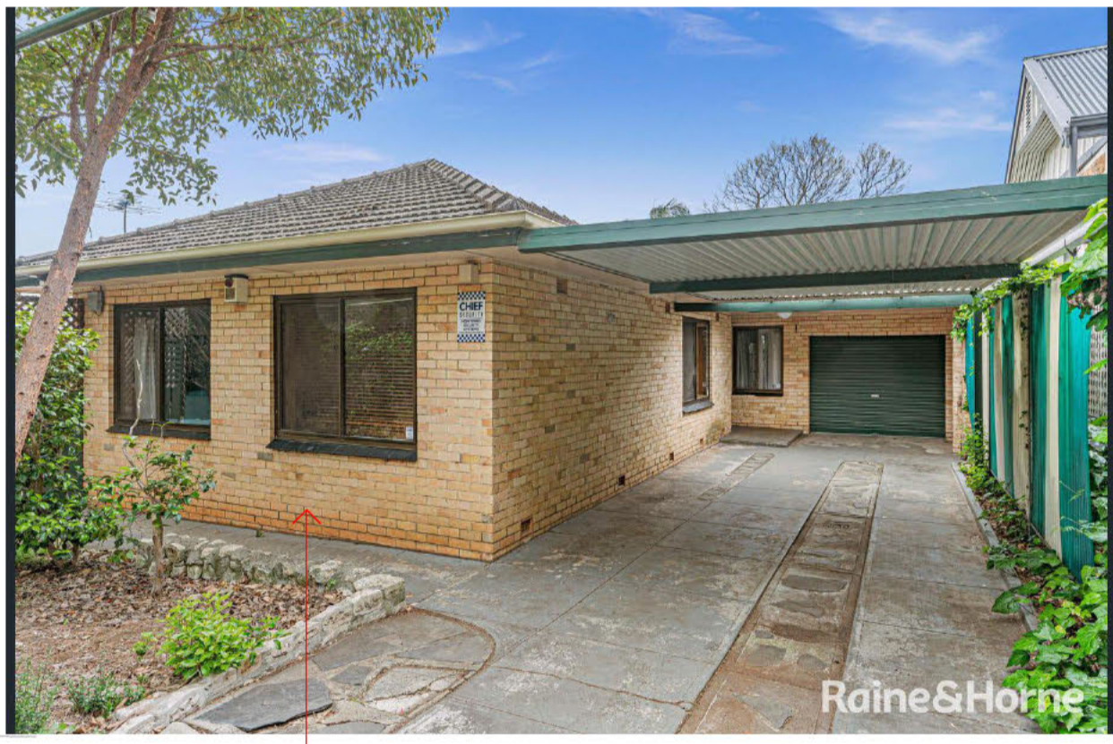
FRONT FACADE OF EXISTING DWELLING PROPOSED TO BE DEMOLISHED
