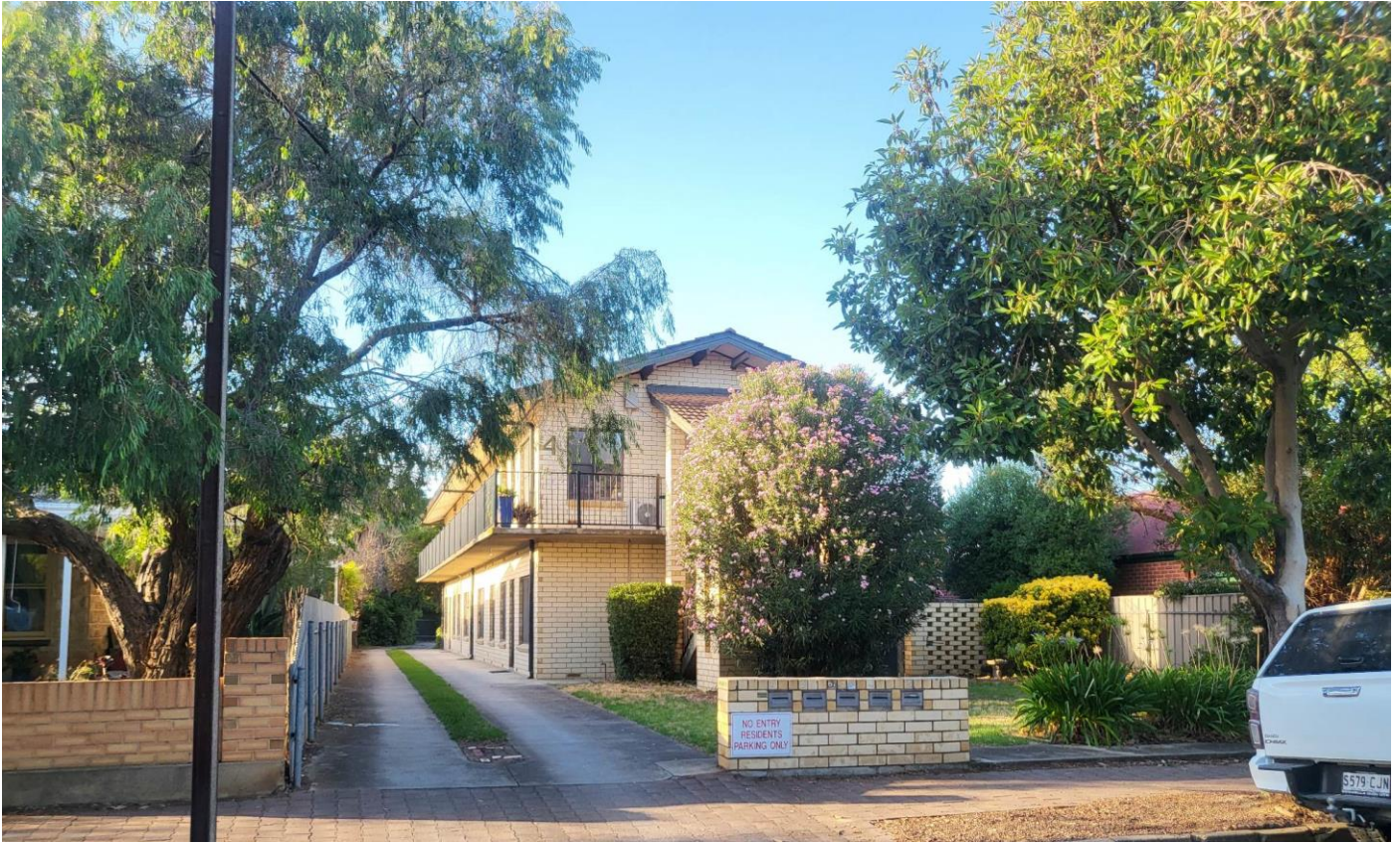
Figure 5: View of the Residential Flat building at 67 Victoria Street.
