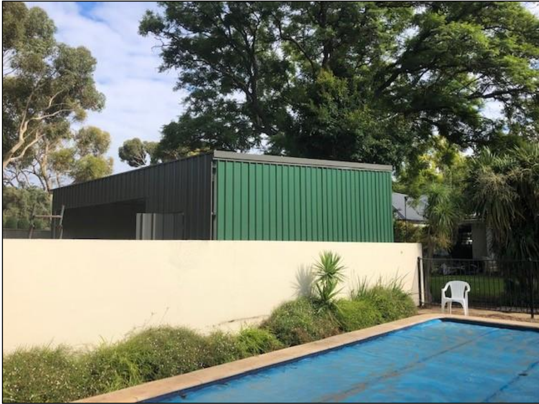
View of the garage from the pool area
