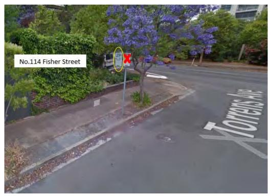
Fisher Street / Torrens Avenue from south east corner Remove existing 2P sign and install sign '2P 8am-5pm Mon-Fri with arrow to left.
