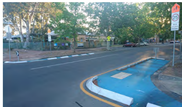
Image 2: An example of pedestrian safety protuberance at the intersection of Surrey Street and Hampton Street South. New kerb, ramps and blue painting treatment to be installed to protect pedestrians and cyclists by reducing the road crossing distance.
