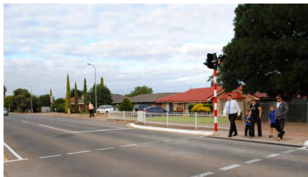
Image 1: An example of the pedestrian crossing point with protuberance, linemarking and flashing lights. Image sourced from: http://www.playford.sa.gov.au/page.aspx?c=14950
