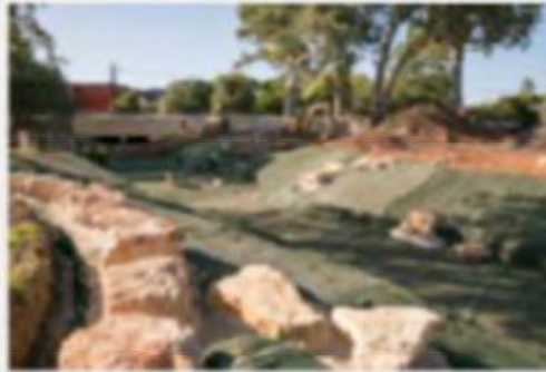
Brownhill Creek Upgrade Pyramat and Stepping Boulders January 2019
