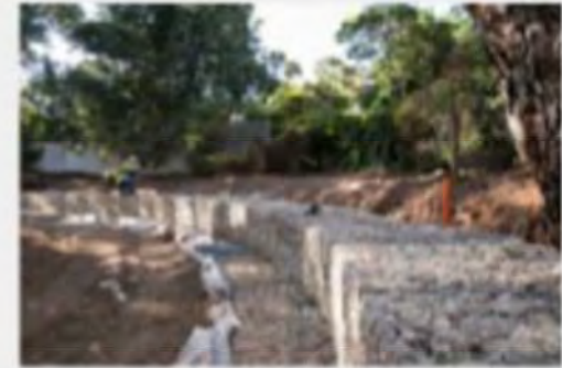
Brownhill Creek Upgrade JWS Morris Gabions January 2019
