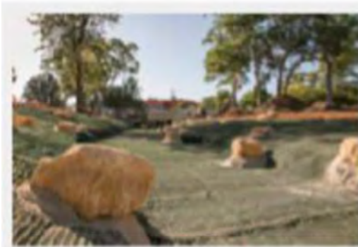
Brownhill Creek Pyramat and Stepping Boulders January 2019
